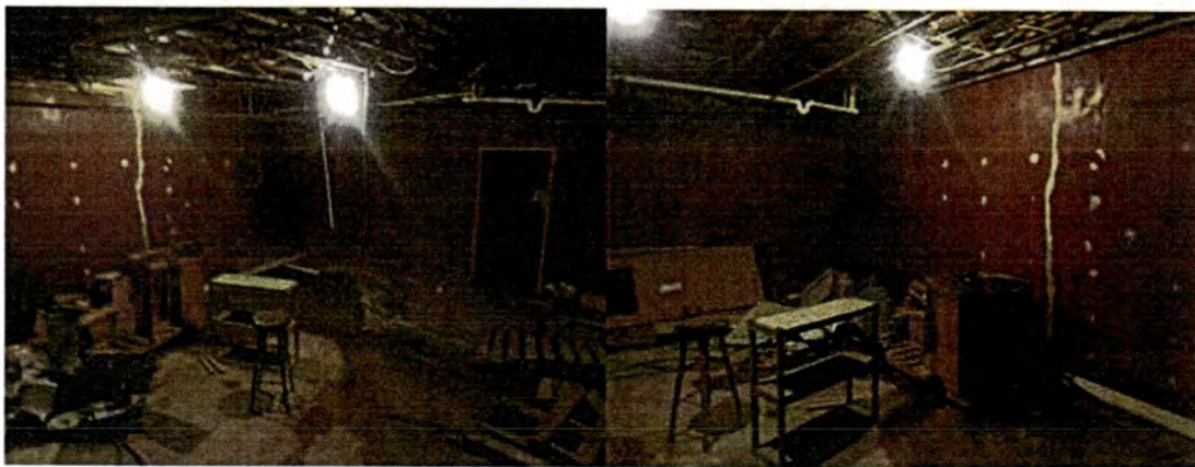
Interior Subject Property Basement
