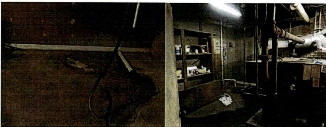
Interior Subject Property Basement
